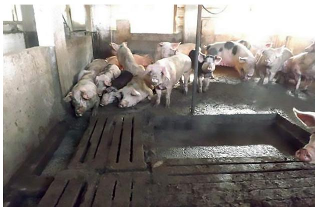
**Figure 1:** Non-compliant floors: cracks and “holes” in breeders and fatteners areas.
